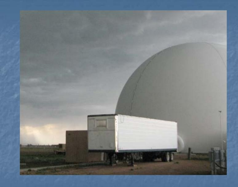
Offset feed antenna installed in spring 2008. Design provides improved cross-pol isolation and reduced sidelobe levels. Main reflector diameter is 8.5 m; 3 dB beam width is 1.0 degrees.
